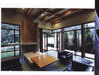
this context. For instance, part of the roof and the north facade have been made from glass to show the imposing 'chasm' staircase to full advantage. By using PSL (parallel strand lumber) wood – technically modified wood – the architect was able to achieve large spans with a minimum of support. "This may be the biggest cantilever in the world for a beam of wood laid sidesways," Julian Jacobs says.
