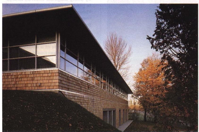
Jacobs describes the construction as 'vertically tripartite', a layering of poured concrete at the first level/basement, steel post and beam perimeter walls at the second level, and glulam trusses spanning a clear 12m in the roof.
