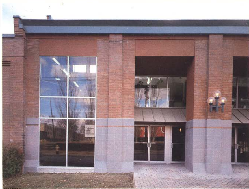
INTEREST WAS CREATED IN THE BLAND EXTERIORS BY SETTING BACK ENTRANCES, WHICH ALSO ALLOWED FOR THE THIRD (FIRE) DOOR.
