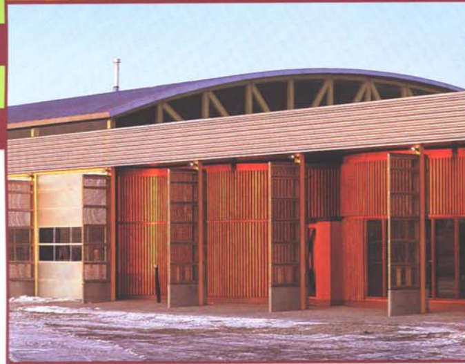
Top: The garage space is vaulted by a curved silver plane supported by bowstring trusses. The frameless glass under the roof gives a sense of levity to the roof.
