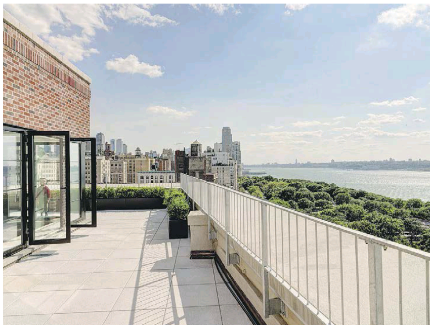
In order to replace crumbling brick on the outside of the apartment facing the terrace, the renovation team had to seek out new brick that exactly replicated the original.
